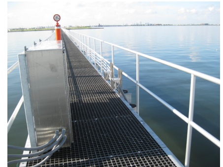
Lakefront Airport New Orleans, Louisiana:
