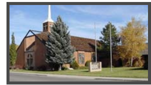
Bethlehem Lutheran Church and School -- energy-efficient electrical systems
