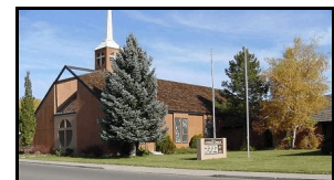
Bethlehem Lutheran Church & School -- energy-efficient electrical systems
