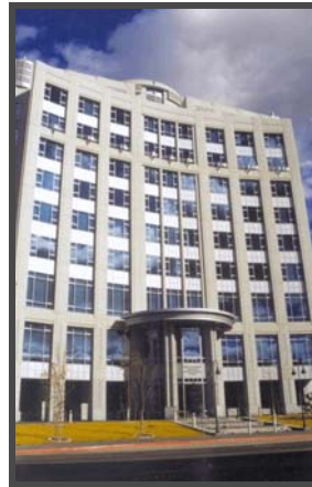
Thompson Federal Courthouse, Reno, NV
